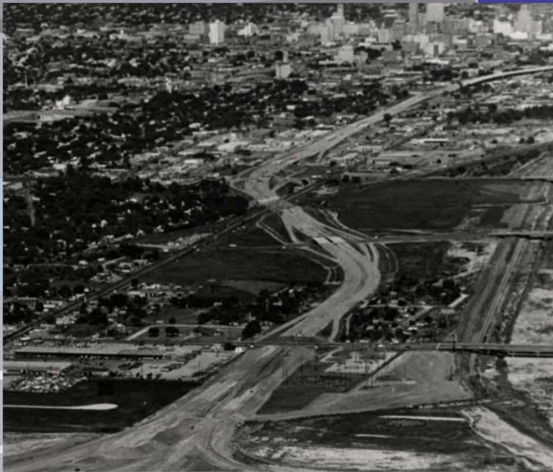
Crosstown grading looking East through Sandtown, 1965 (2)
