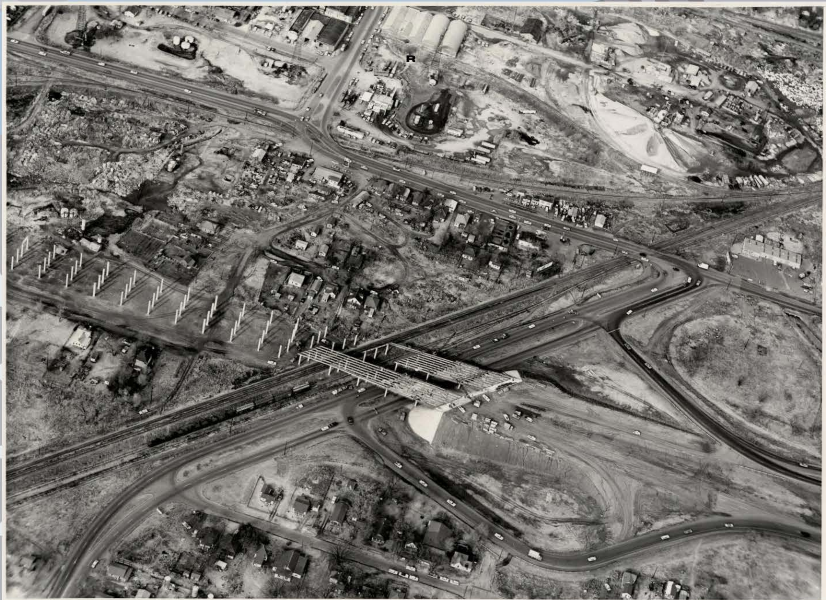
Elevated highway construction through Walnut Grove, 1963 (9)
